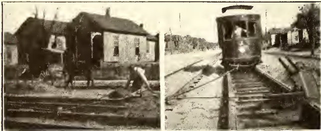
STREET CAR USED TO PULL SCRAPER IN DALLAS, TEXAS
